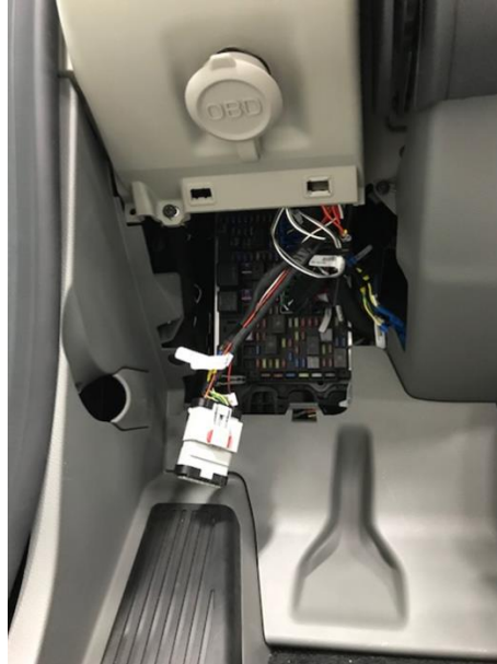
RP1226 Connector Inside the Cab (See “Section 7 Electrical” For More Locations)
